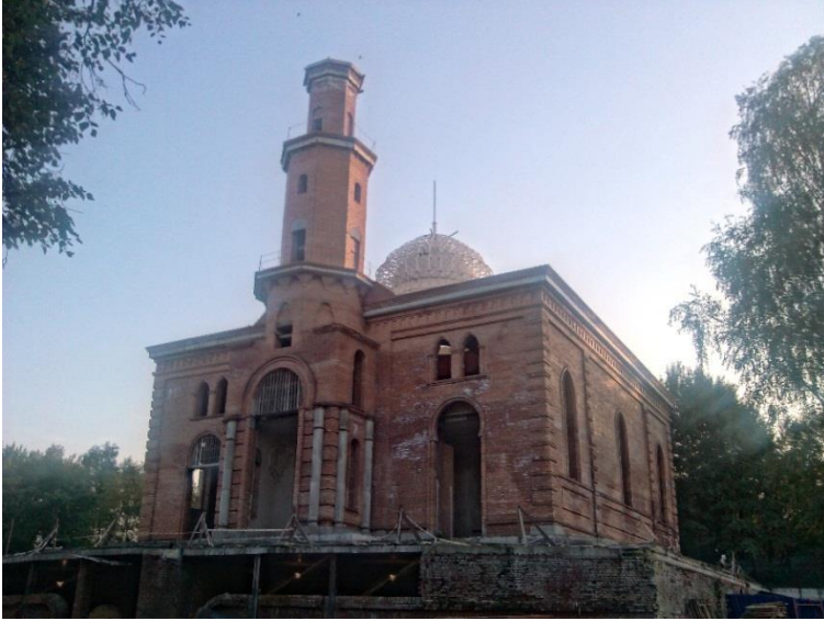
Construction of a mosque 11 Sep, 2014
