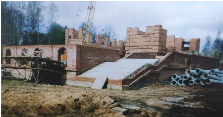
Construction of a mosque April 2005
